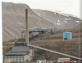
C The coal-fired power station at Longyearbyen
