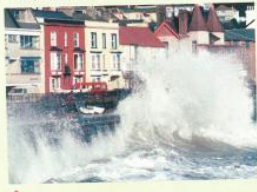
A Sea wall at Dawlish, Devon
