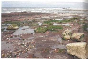
A The breach of the sea defences at Medmerry
