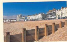
B Groynes at Eastbourne, Sussex
