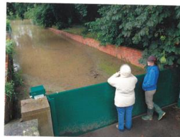
D Flood gate protecting property from the rising River Severn, Deerhurst, Gloucestershire
