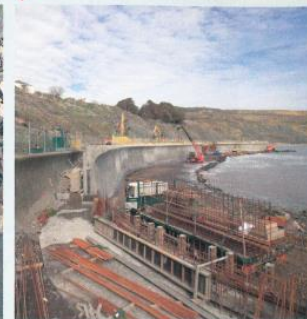
C Phase 4 coastal defence works at Lyme Regis
