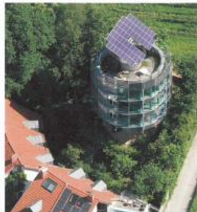
C The 'Heliotrope' rotates to follow the sun
