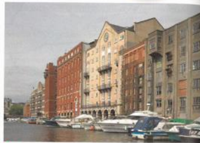
A Warehouses converted into flats along Bristol's harbour front
