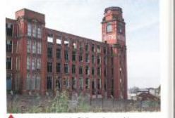
A derelict factory in Oxteth, Lancashire
