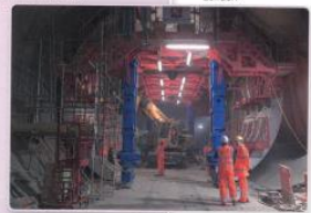
The construction of Crossrail deep below London
