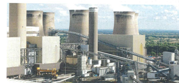
E The Drax power station
