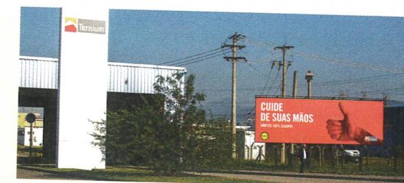
D Ternium steelworks, Sepetiba Bay, Rio
