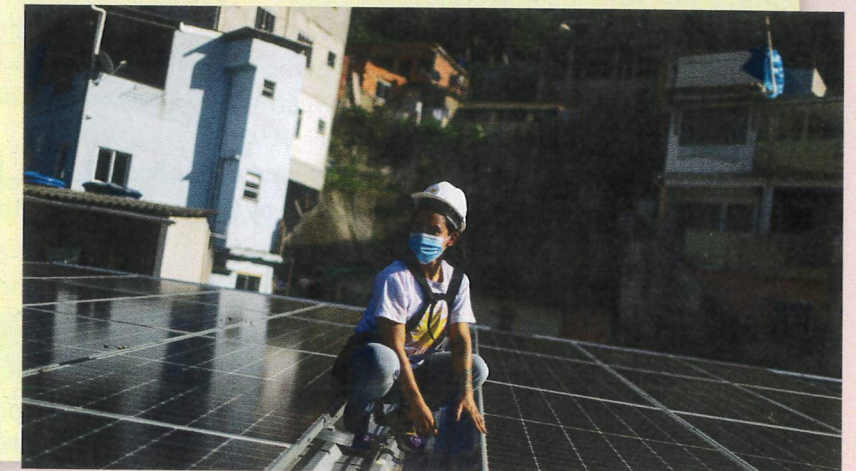
D Solar system installer Natalia Noel Nazario checking solar panels installed in Babilonia favela, Rio
