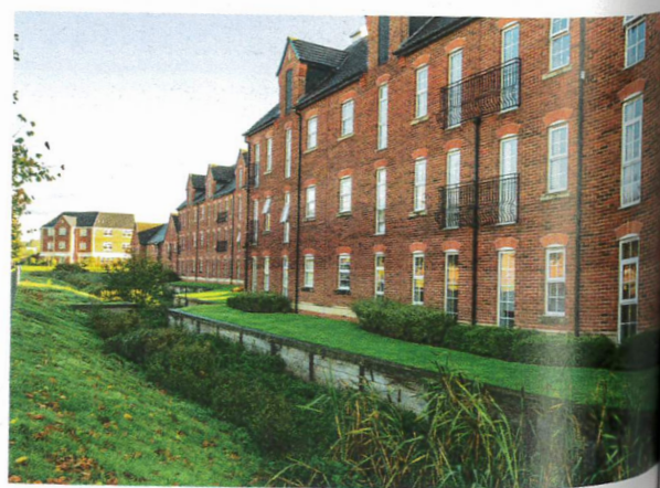
B Sustainable drainage system in Lancashire
